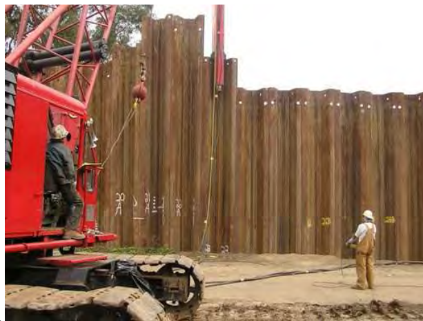
Figure 4.1 Construction of sheet pile wall. From Associated Pacific Constructors(2010).
