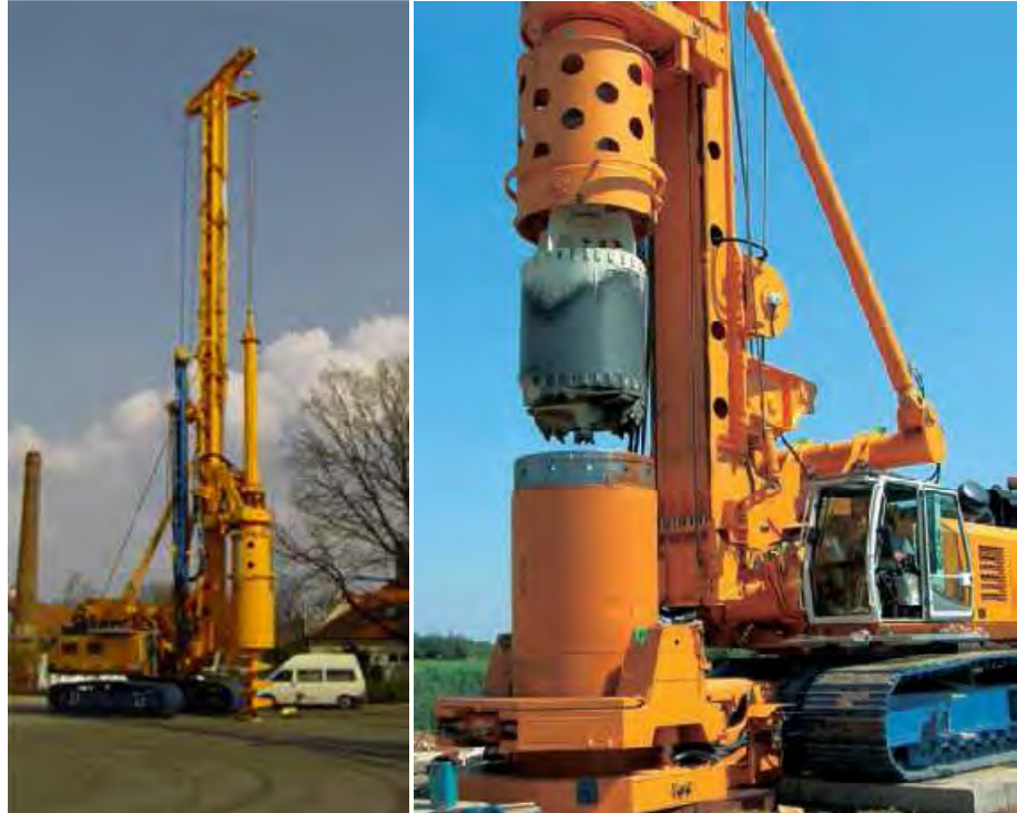
Figure 4.21 Left: Bauer dry drilling unit; right: Bauer dry drilling unit fitted with casing oscillator.
