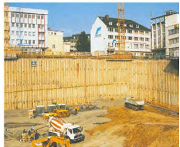
Figure 4.2 Construction of secant pile wall. From Bauer Group (2010).
